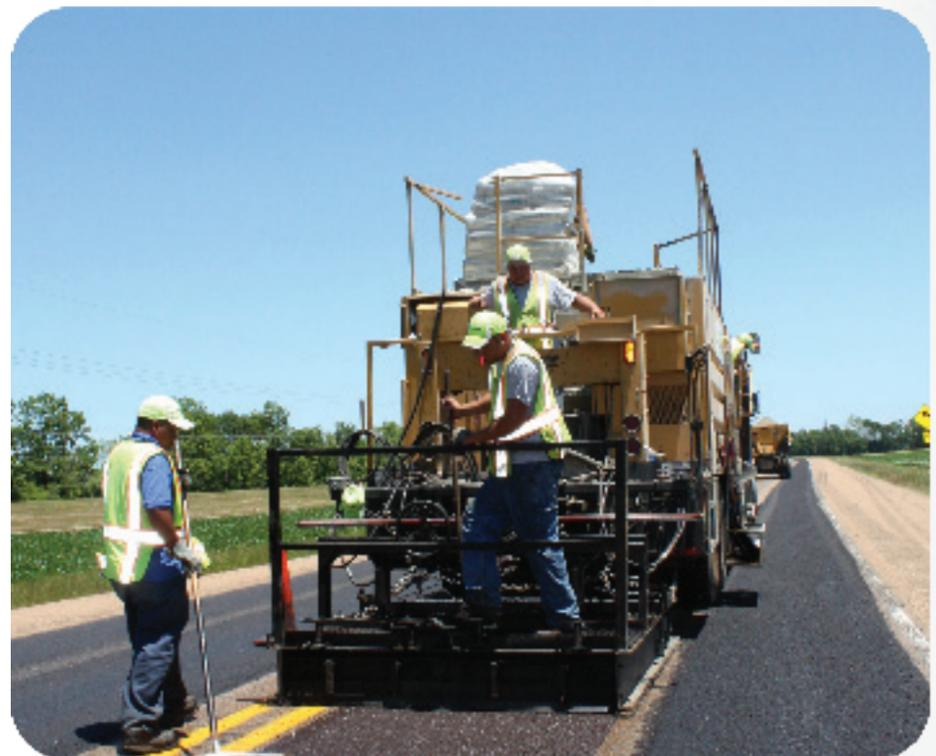
Vance Brothers uses a rut box attached to a Bergkamp Mobile Mix Paver to fill wheel ruts with micro surfacing.
