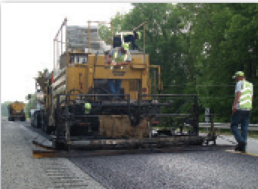
*Bergkamp mix paver applies micro surfacing over entire 12-foot lane width in a single pass.*
