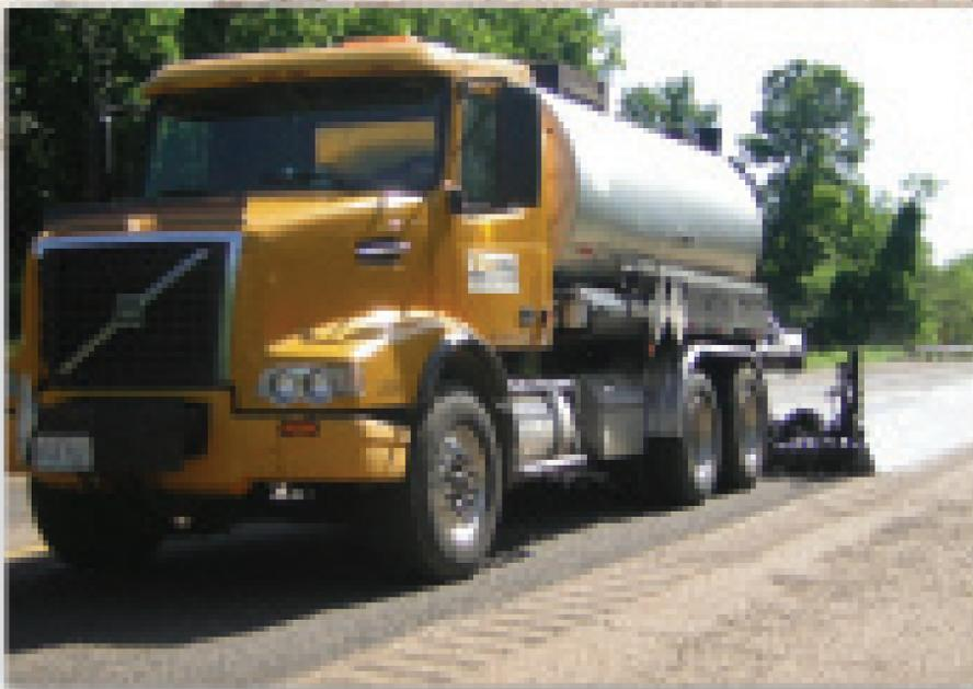
*Contractor's Volvo distributor truck sprays SBR latex-modified CRS2-P emulsion for the chip sealing treatment.*
