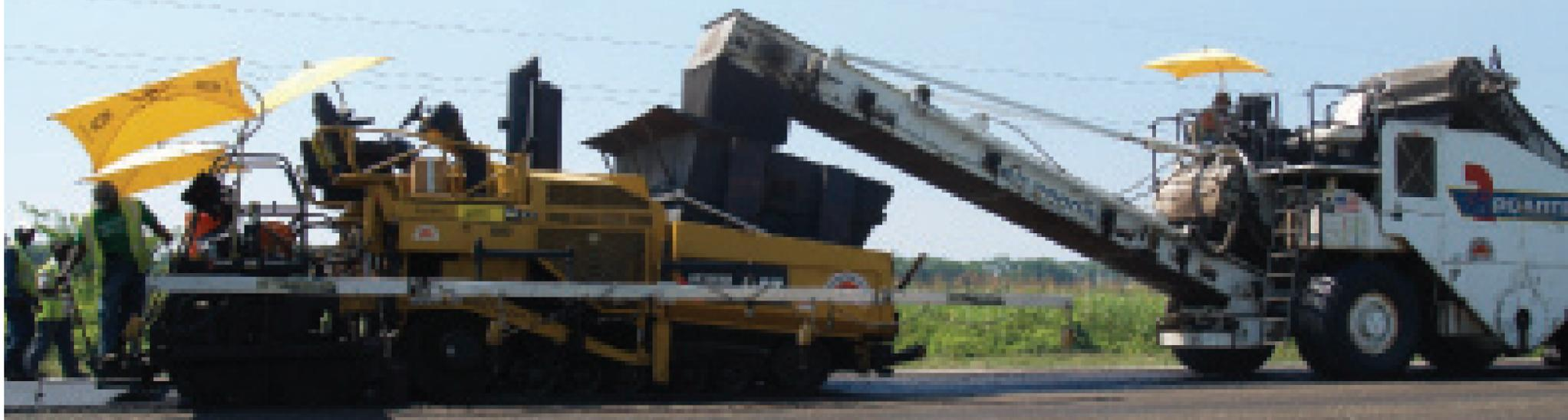
Supported by a ROADTEC Shuttle Buggy, a CAT 1055D paver places a 1-1/2-inch Superpave asphalt wearing course.
