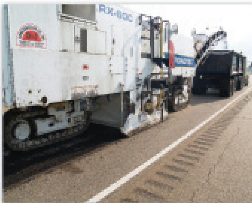
D&J Construction Company's ROADTEC RX60C mills off ½-inch of existing pavement prior to chip seal placement.
