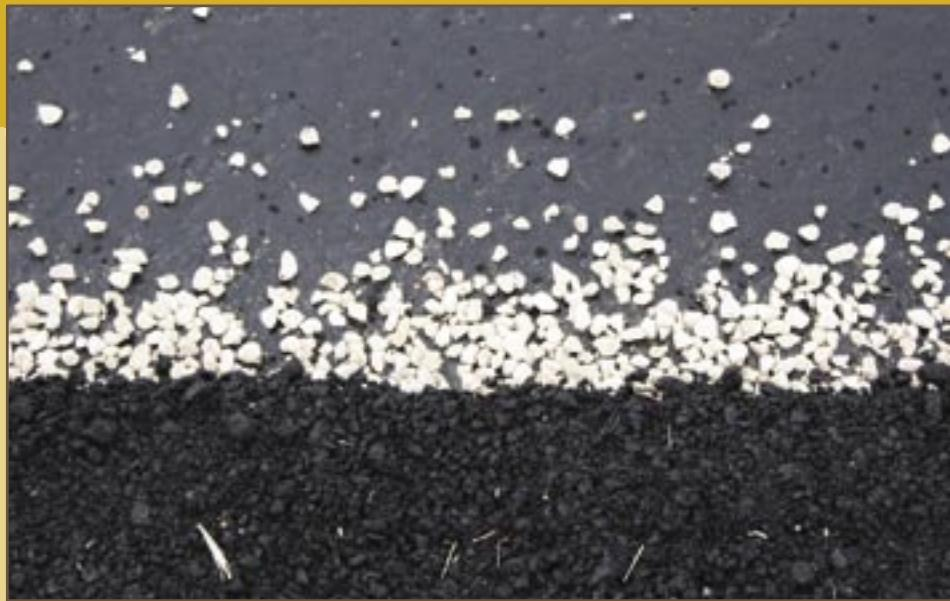
Top: Ahead of paver, Etnyre ChipSpreader broadcasts aggregate on cationic high-float asphalt emulsion to create underseal designed to bond overlay to existing pavement.
